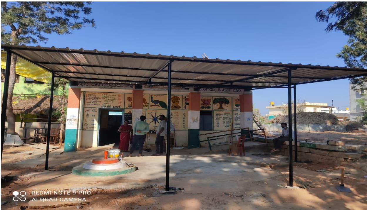
Photos: School Shed Constructed by CSA Volunteers:
