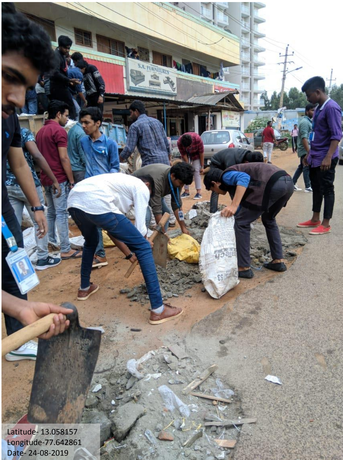
Students in potholes repair work
