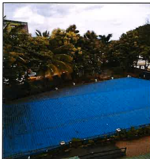
Rainwater Harvest Tank
