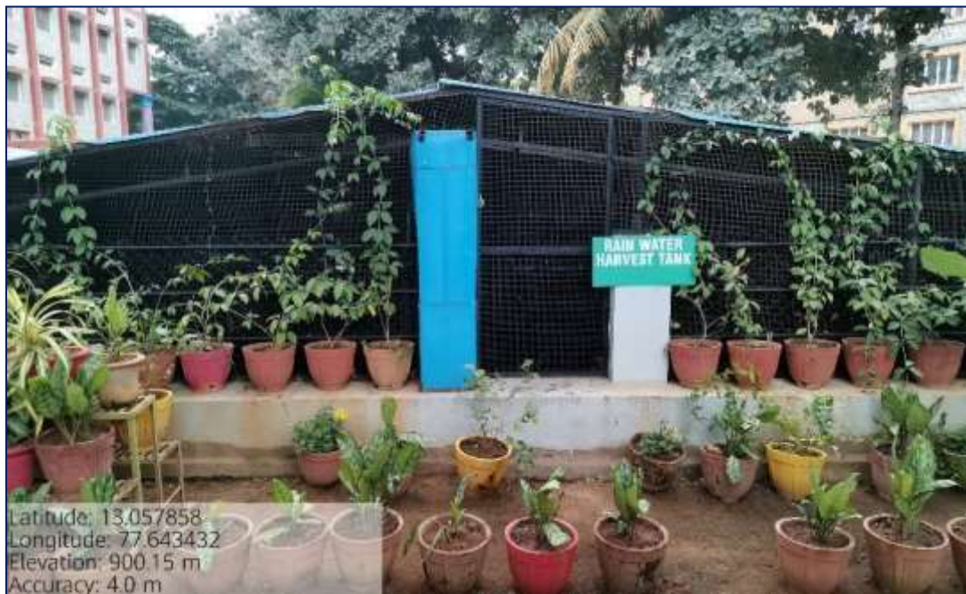
Figure 6: Rainwater harvesting tank near main block
