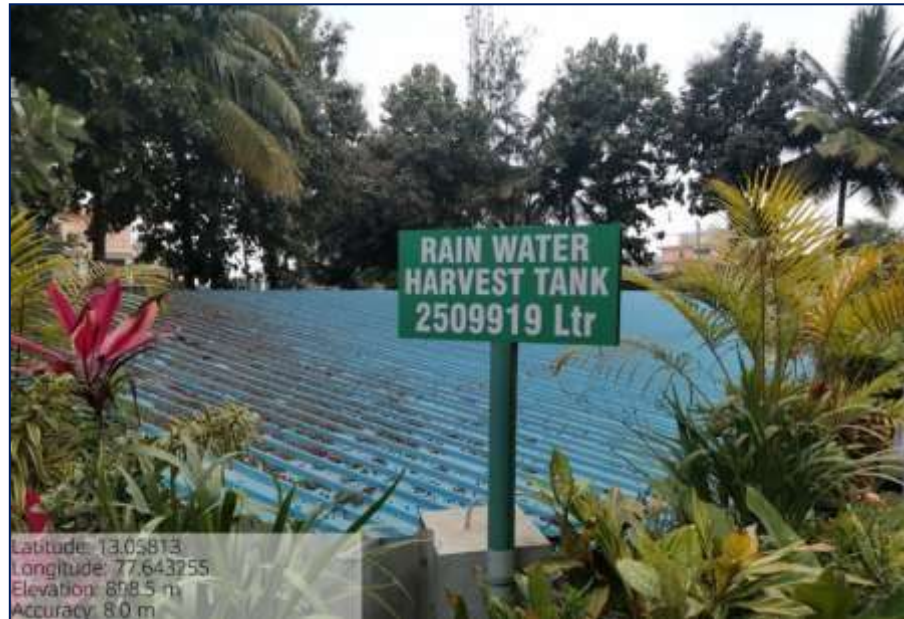
Figure 5: Rainwater Harvesting Tank of 2.5ML Capacity
